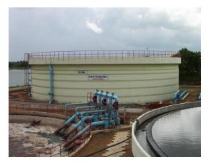
TNPL put-up closed high rate bio-methanation reactors (biogas plant) in phased manner during 2003, 2008, and 2017 to treat high COD bagasse wash wastewater under waste to energy concept. In the reactor organic pollutants present in the wastewater are converted into methane and captured & used as in-house renewable fuel in lime kiln to replace furnace oil.
