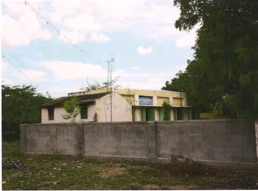
Photograph of Murthypalayam Panchayat Union Primary School compound wall (View from outside premises)
