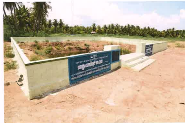
4. Close view of the constructed parapet wall
