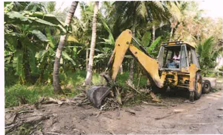
2. Debris being collected by JCB
