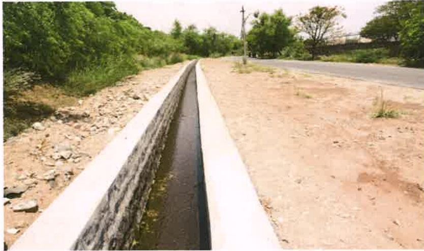
Overall view of storm water ravine constructed at Murthypalayam village
