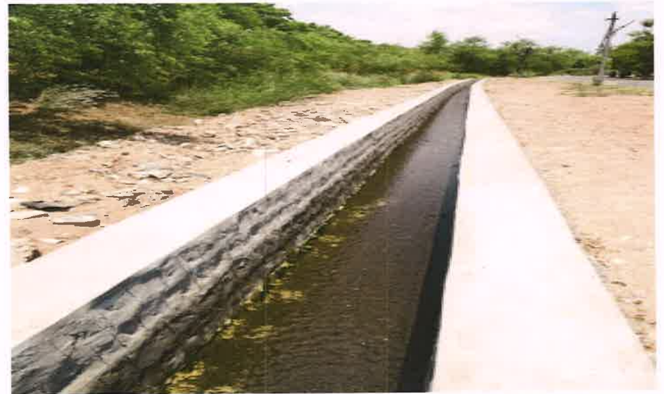
Close view of the storm water ravine constructed at Murthypalayam village
