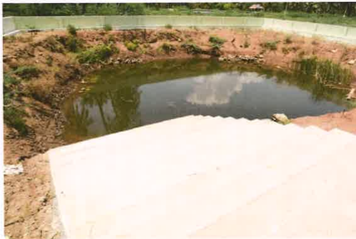
3. Approach steps to the well
