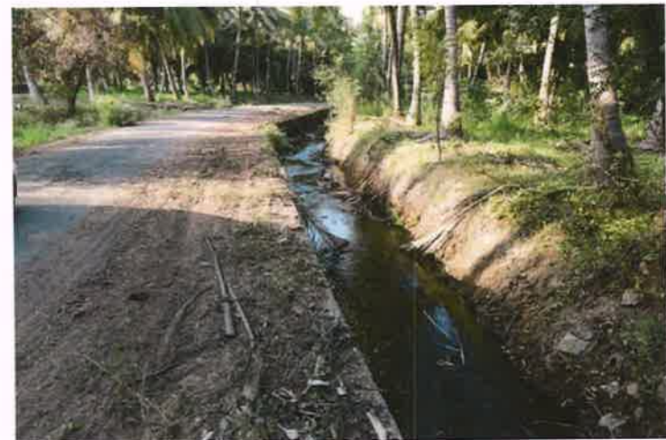
4. Cleaned road from Moolimangalam to Murthipalayam
