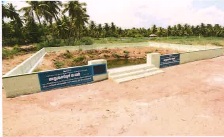
1. Overall view of parapet wall constructed
