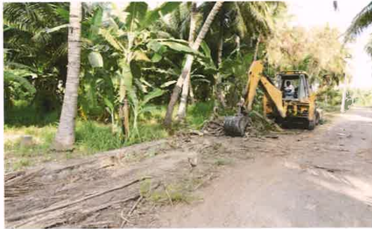
1. Bushes being cleared by JCB
