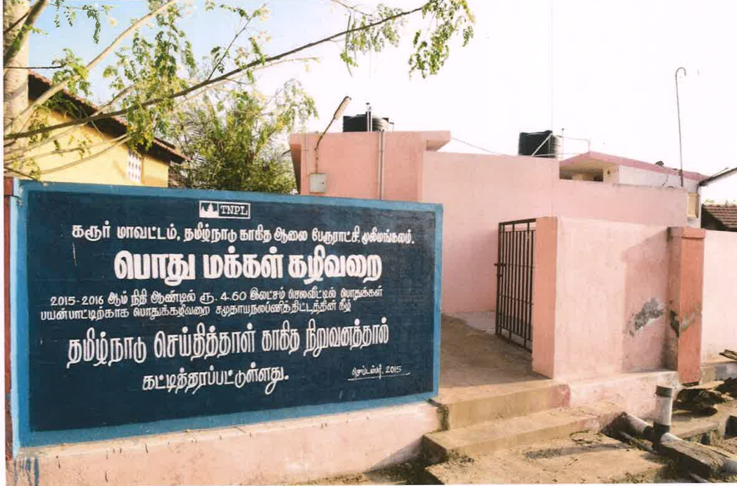
Public toilet at constructed at Moolimangalam
