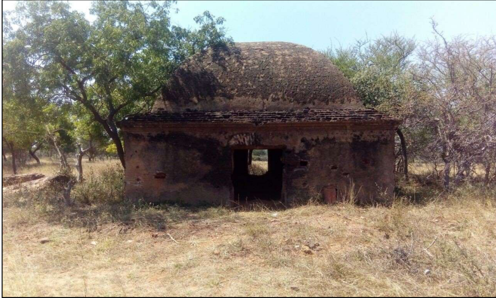
Fig. British Period Ammunition Structure found nearby TNPL Unit-II
