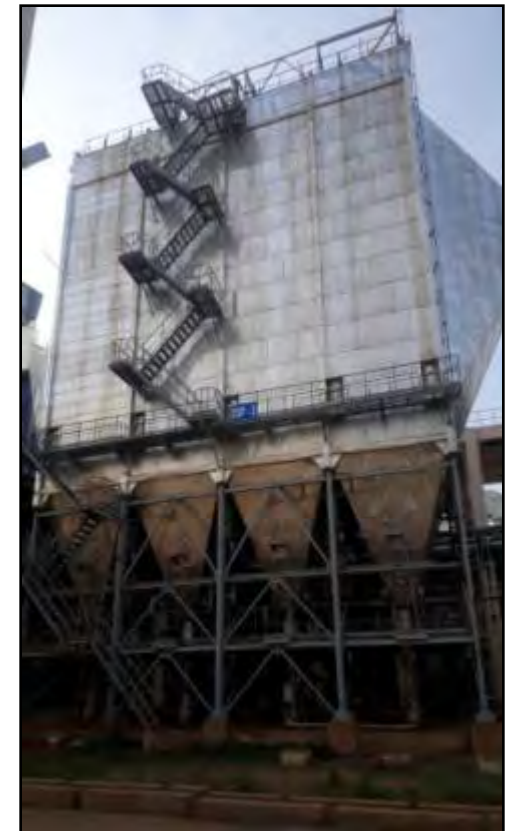
Power Boiler Electro Static Precipitator (ESP) – 1&2
