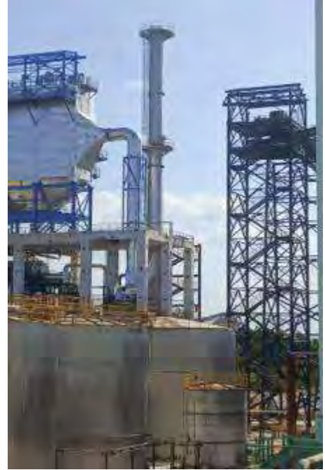
Lime Kiln Stack – 54.8 m height
