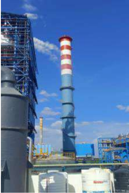
Chemical Recovery Boiler Stack – 90 m height
