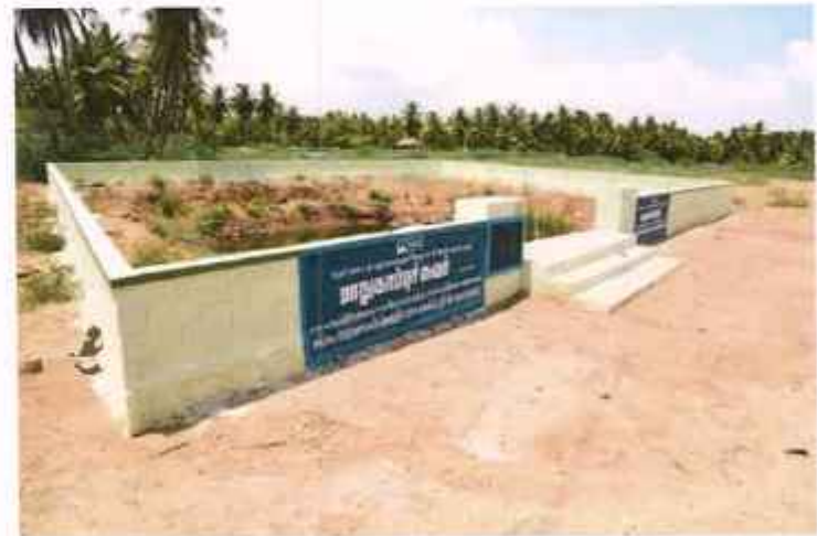
4. Close view of the constructed parapet wall
