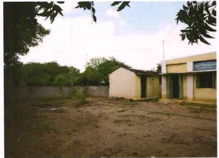
Photograph of Murthypalayam Panchayat Union Primary School compound wall (View from inside premises)
