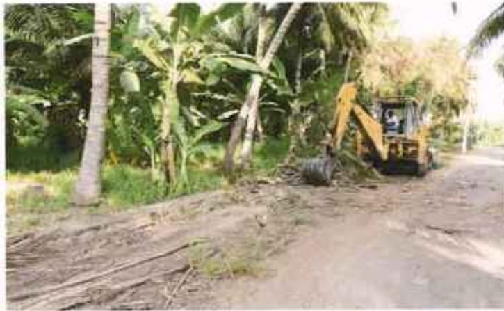
1. Bushes being cleared by JCB
