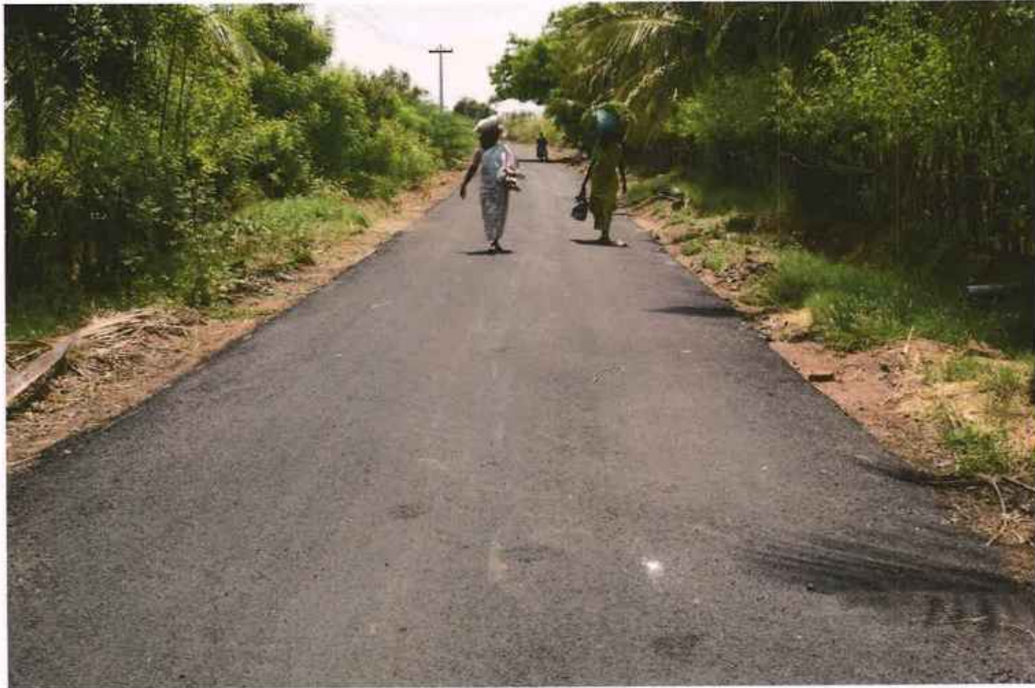
View of Black Topped road repaired and relayed by TNPL at Punjai Thottakurchi village
