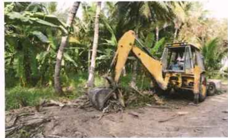
2. Debris being collected by JCB
