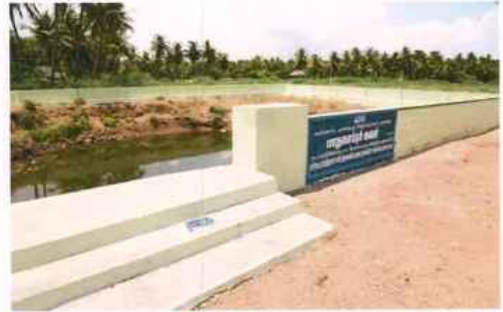
2. Well entry point
