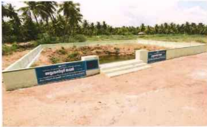
1. Overall view of parapet wall constructed
