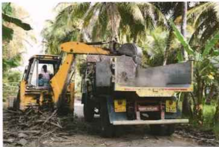
3. Cleared bushes and debris are loaded in tipper for disposal
