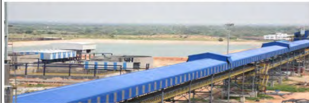
Closed hoods for coal conveyors
