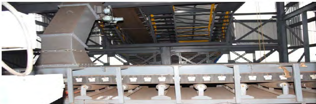
Closed transfer of coal between conveyors
