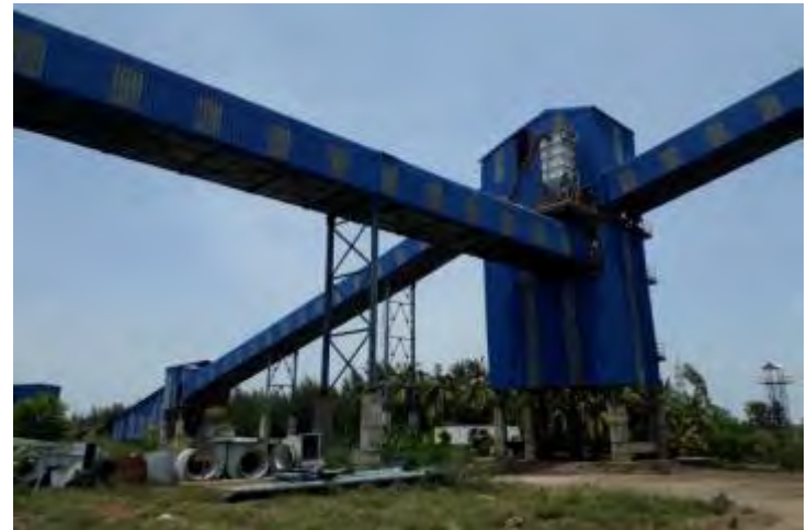
Closed hoods for coal conveyors
