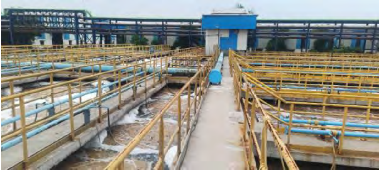
MOVING BED BIOFILM REACTOR (MBBR)
